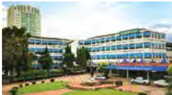
Srinagarindranusorn Building Khon Kaen University
