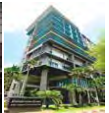
Computer Bldg. Kasetsart University
