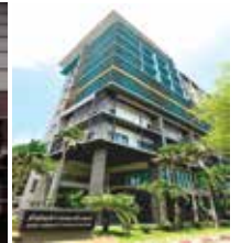
Computer Bldg. Kasetsart University
