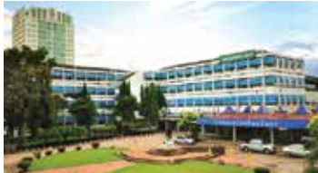
Srinagarindranusorn Building Khon Kaen University
